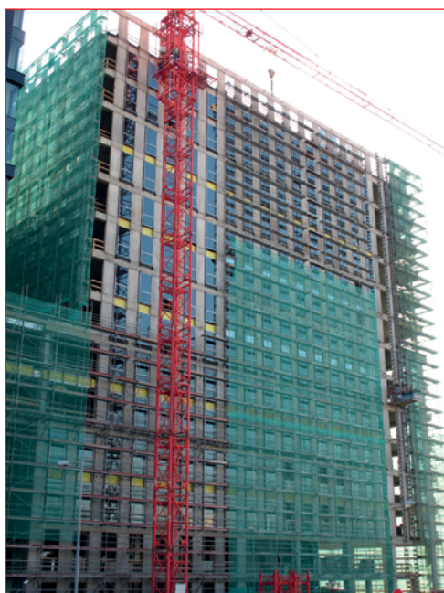
Budowa Quattro Business Park - Kraków
