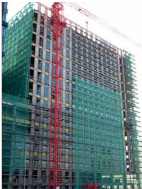
Budowa Quattro Business Park - Kraków
