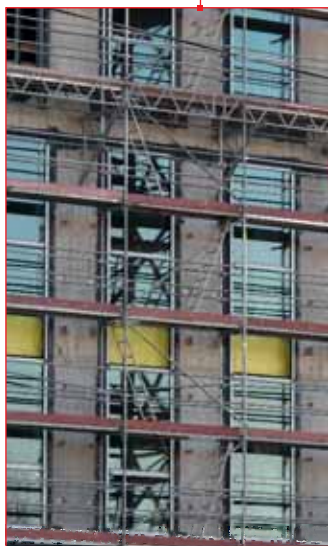
Budynek Quattro Business Park - Kraków
